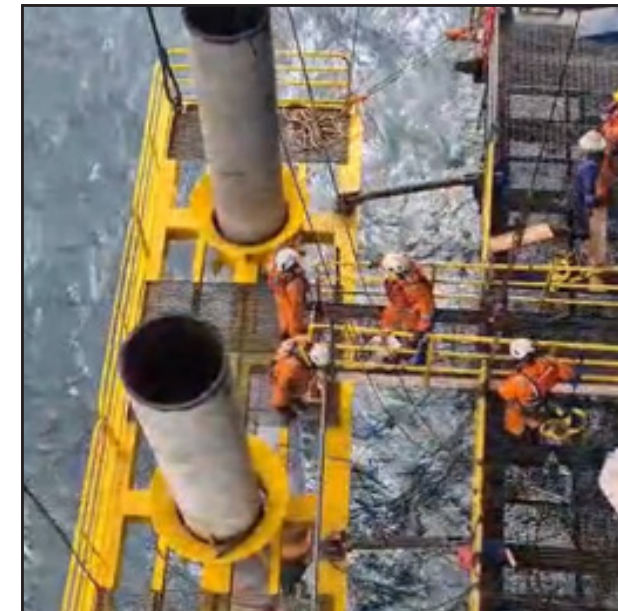
Conductor Installation Template
