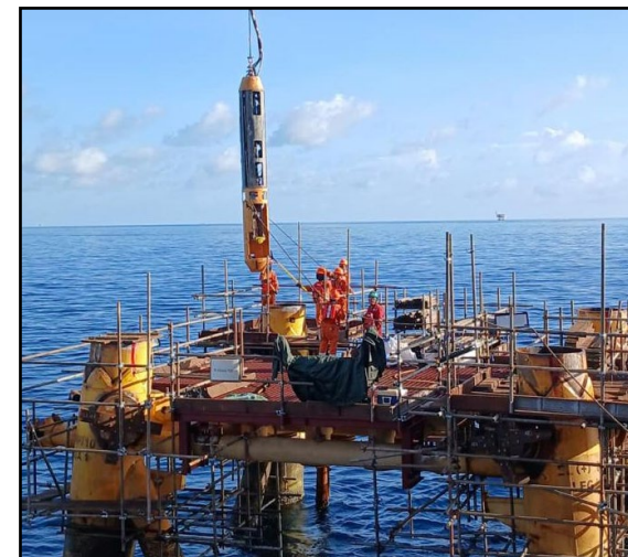
Jacket being lifted after completion of abrasive cutting
