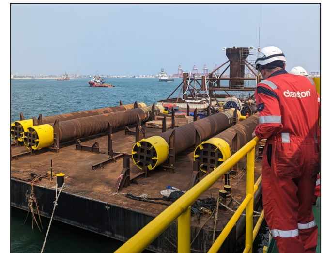
Four of the Abrasively Severed Piles in Transport Holding Frame
