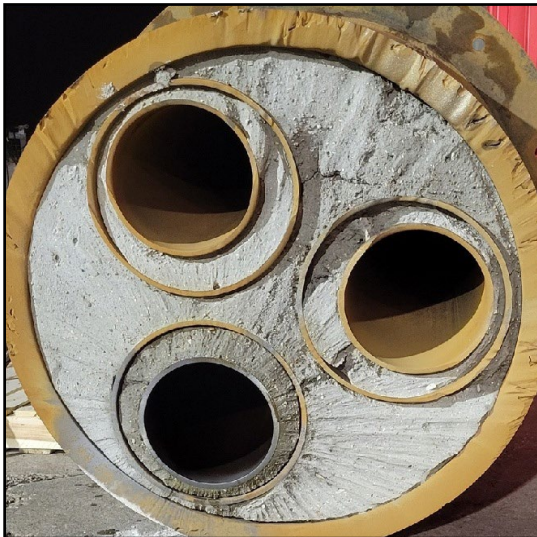
Completed cut on triple bore well
