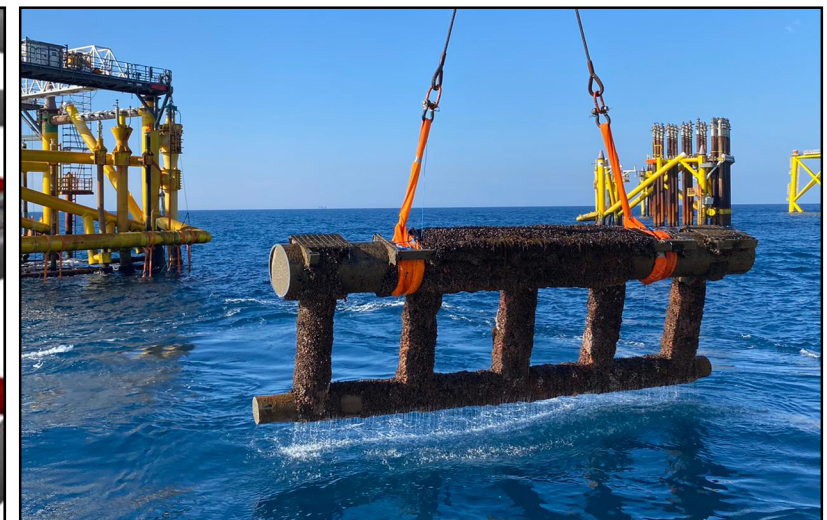
Removed structure section cut with Diamond Wire Saw
