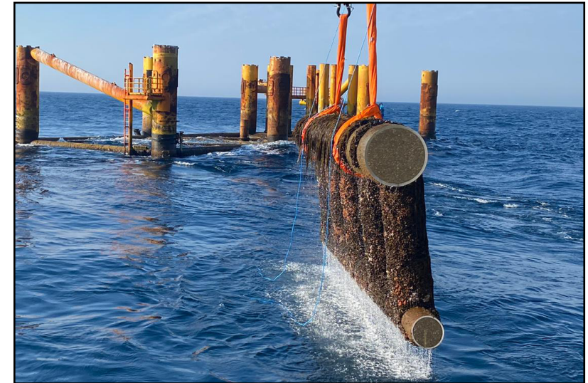
Removed structure section cut with Diamond Wire Saw
