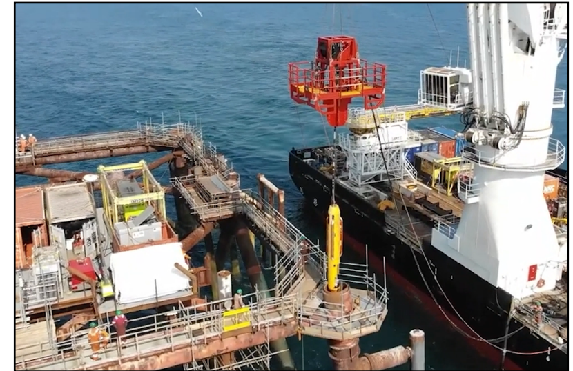
Claxton Internal Pile Cutter deployed into Jacket Leg
