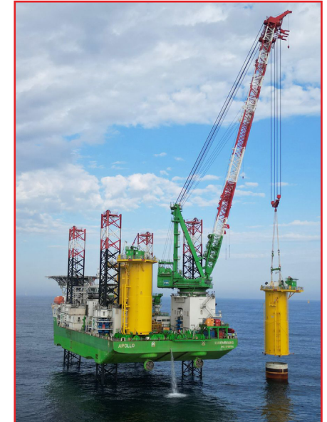
Installation of the transition piece onto a monopile, post cleaning project.
